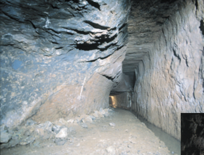
Ginzan Sakunouchi. Traces of Early Modern(right) and Modern(left) digging at Ôkubo-mabu. (South valley of Mt Sennoyama)
