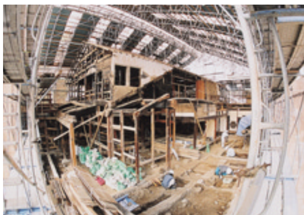
Restoration and repair work
