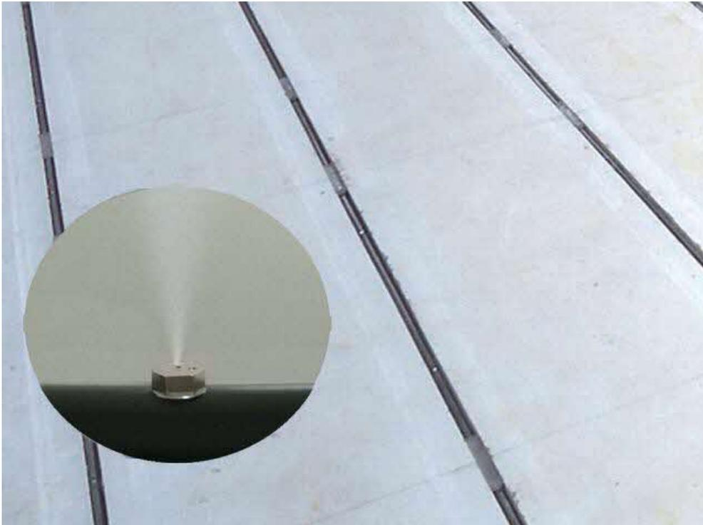
By sending air from a special nozzle at 50 times the pressure of a conventional blower, it raises the fermentation temperature quickly and reduces the processing period dramatically. It can be installed in existing facilities to help reduce turning work as well as foul odors.
