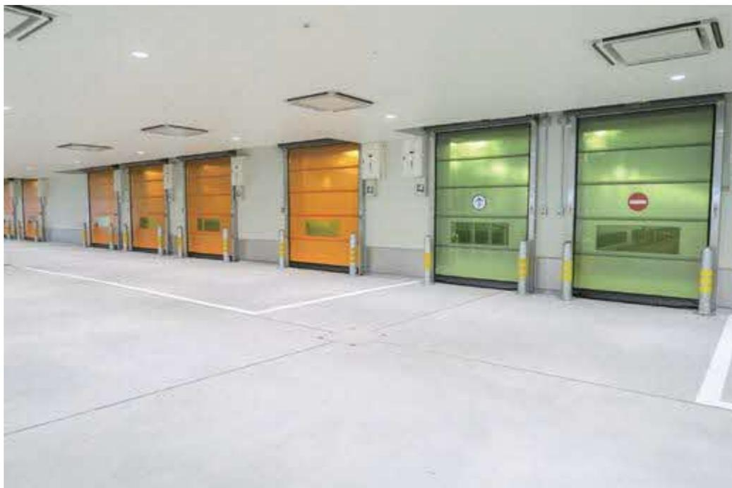
Thanks to its high airtightness and high speed opening and closing, the high speed sheet shutter “happy gate monban” dramatically improves insect repellence, dustproofing and cold protection as it is installed at plant entrances and partitions. Effective in improving quality and workplace environment. It promotes CO<sub>2</sub> reduction through energy saving.
