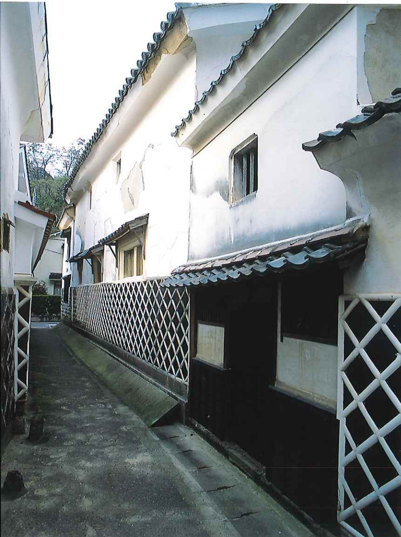
Yunotsu. Cargo ship merchant's houses as part of the historic townscape, seen from southeast.
