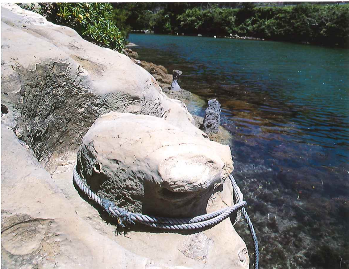
Okidomari. The mooring device carved out of the rockbed, seen from west.
