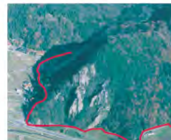
Photo 5. Iwami-jō Site (from above)
